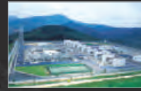
Electro Electric Systems Division
